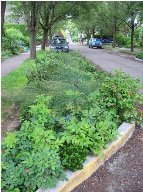
✓ Rain gardens reduce the stormwater/rainwater runoff into storm sewers and create attractive landscaped streets with defined parking areas.
